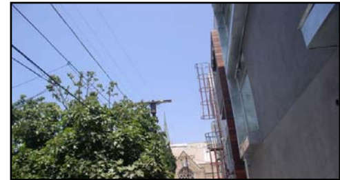
The high voltage lines in relation to the building
